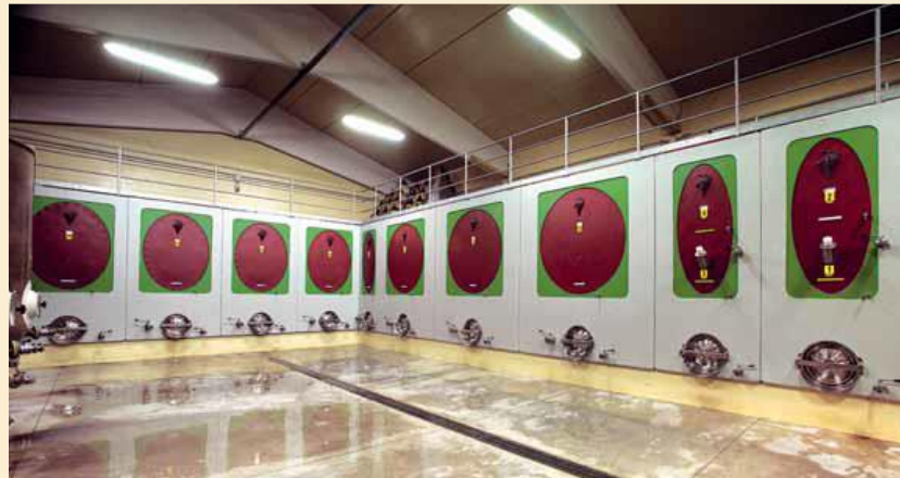
Serbatoi in cemento
