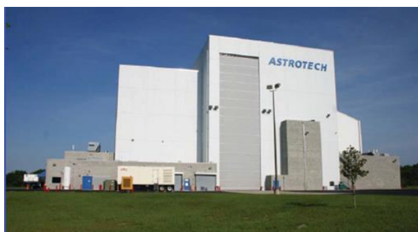
Figure 9-3: Astrotech Space Operations Spacecraft Processing Facility
