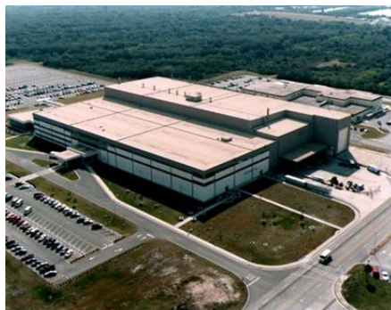
Figure 9-2: NASA/KSC Space Systems Processing Facility (SSPF)
