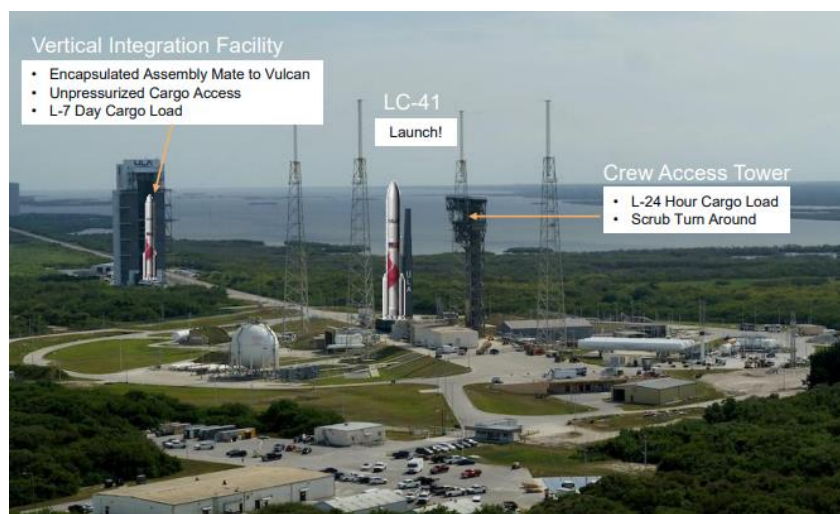
Figure 9-7: SLC-41 Launch Pad
