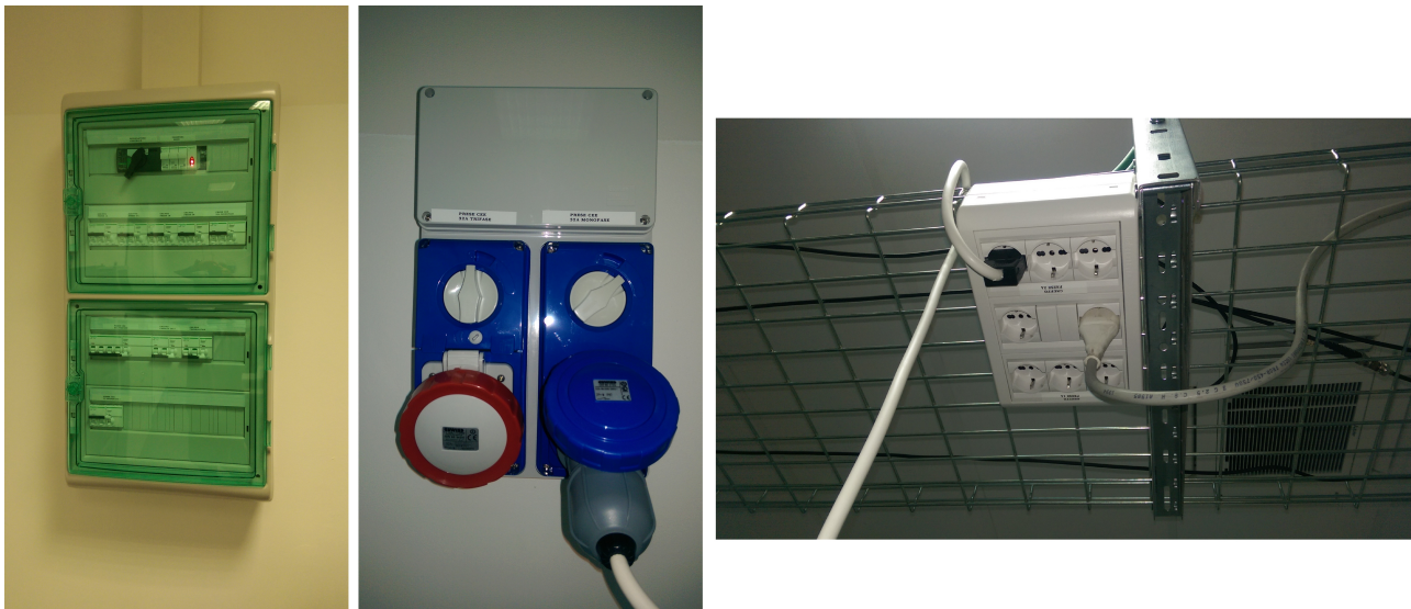
Figura 3: power plant reserved to lasers and instruments. From left to right: electrical cabinet, industrial-type socket, roof shelter sockets.
