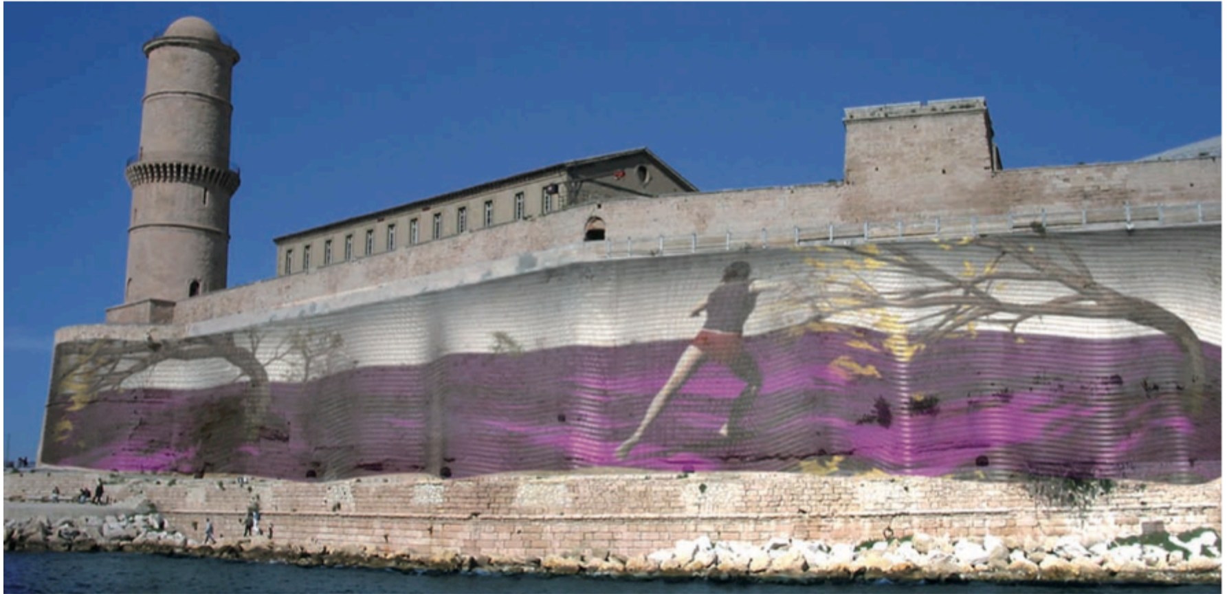
Exterior Daylight Programme AC, see p. 32. "A new technique combining metal mesh shading and LED video transmitters used to create a gigantic screen that is visible in daylight. New technology made available to European and Mediterranean artists" – Image courtesy of N+H Corsica
