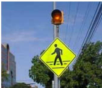
Figure 11-6. Photo. Flashing beacon treatment in Austin, TX.
