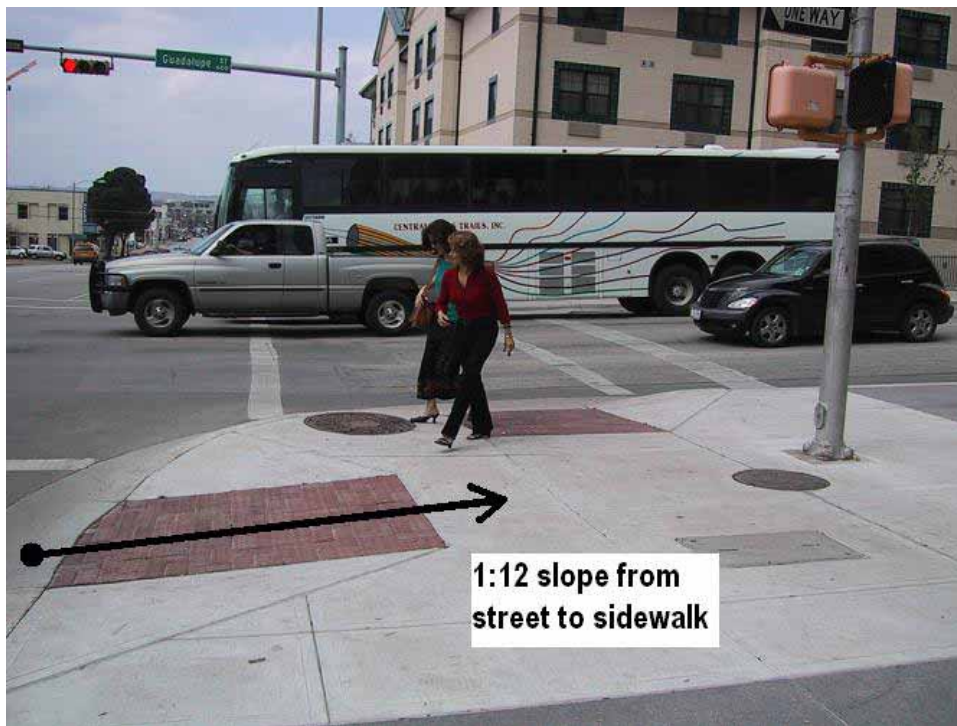
Figure 8-15. Photo. Perpendicular curb ramp.
