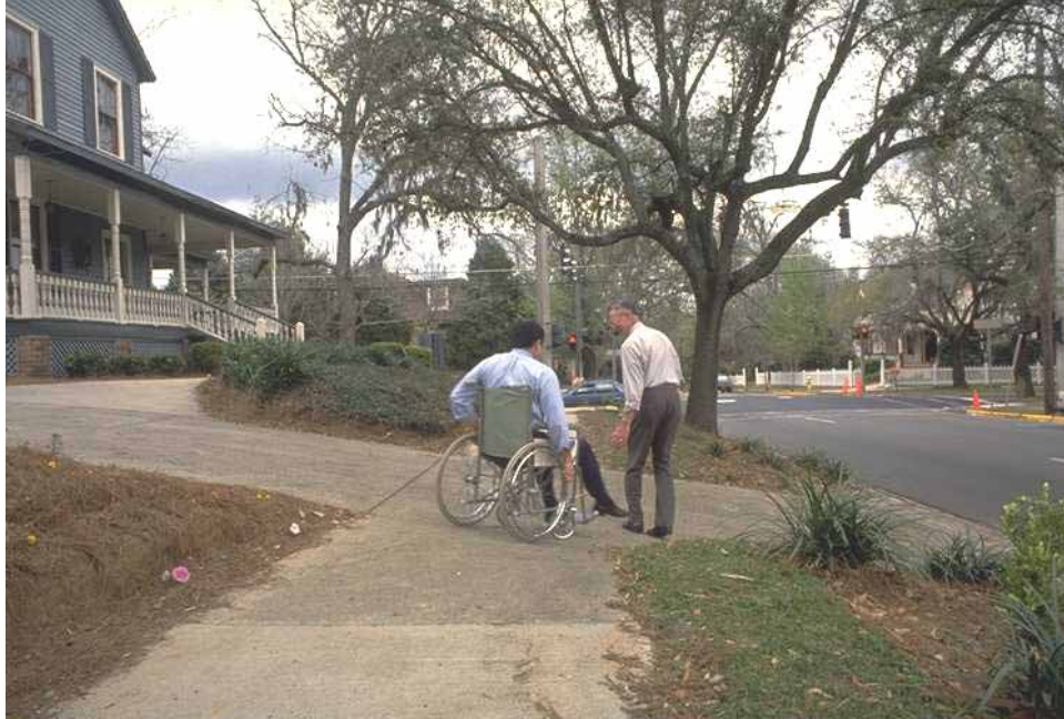
Figure 8-9. Photo. Driveway slopes should not encroach into the sidewalk.
